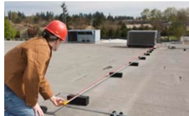
Measuring long conduit runs.
