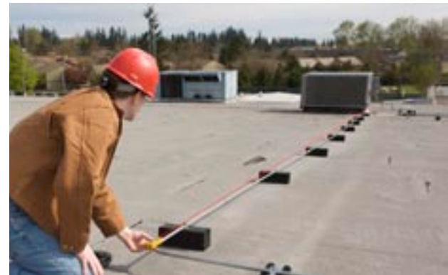
Measuring long conduit runs.
