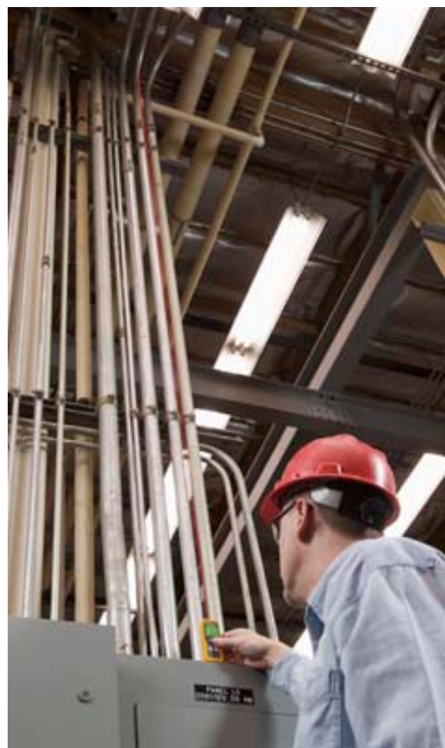
Measuring height to tall ceiling.
