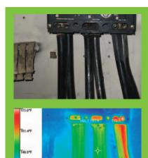
The connections on this evaporator pump read over 50 degrees hotter on phase C.
