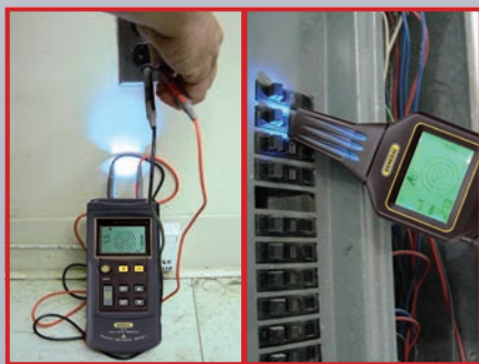
Locating a circuit breaker
