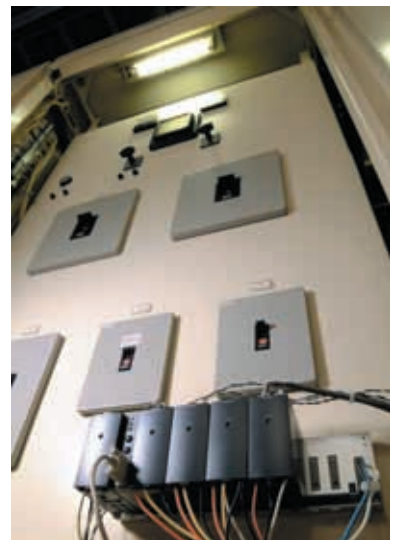
For Monitoring Power Consumption
