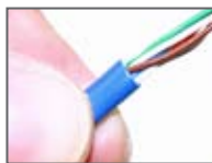
Flatten all pairs together
