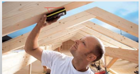
Carpenter – overhead inclination measurement with the 360° tilt sensor
