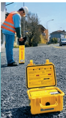
Locate the buried service
