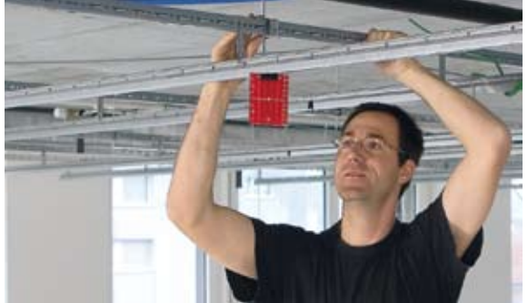
Constructing walls and ceilings
