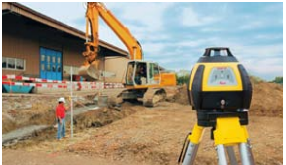
Controlling depth for excavation
