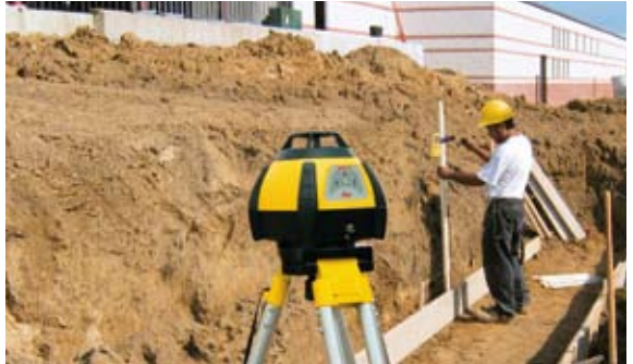
Setting out foundations and walls
