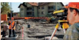
As-built elevation checking, grade checking, area leveling, volume determination of earth/dirt moving operations
