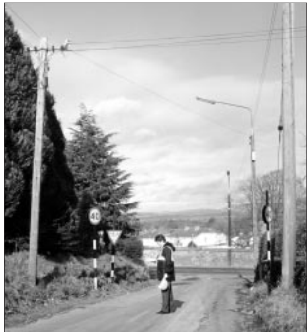
The CHM2000 being used to measure the height of the overhead cable
