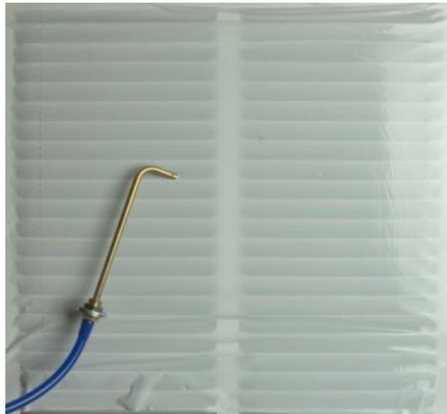
Figure 21: Insert the blue tube into a supply register closest to the air handler
