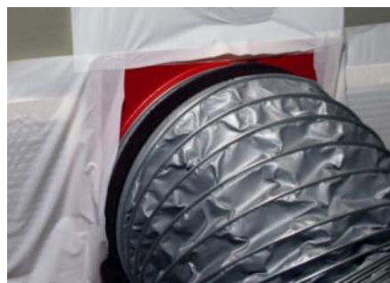
Figure 23: Flex Duct connected to the Flange.
