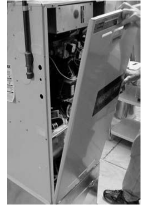
Figure 25: Preparing to connect to ducts via air handler
