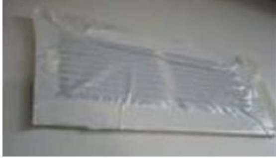
Figure 26: Seal all supply and return registers with Grill Mask
