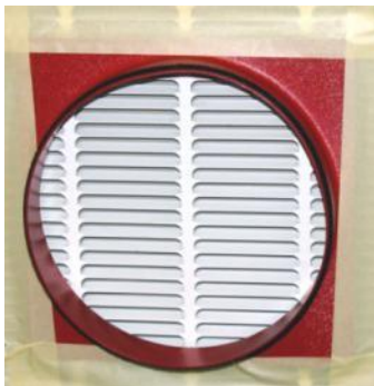
Figure 24: Flange taped onto a return register before attaching the Flex Duct
