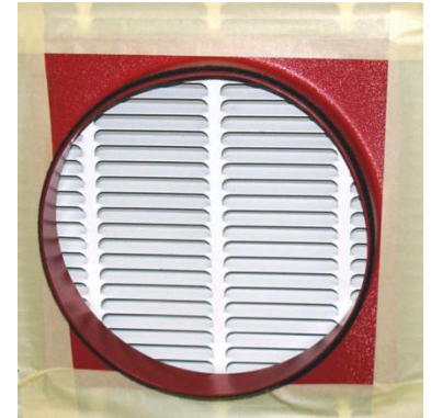
Figure 23. Flange taped onto a return register before attaching the Flex Duct
