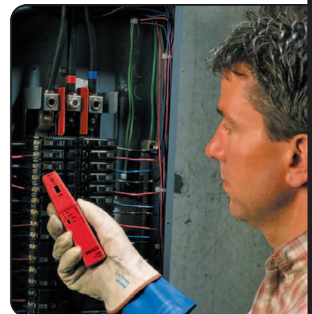
Find the right circuit breaker, sort and trace wiring
