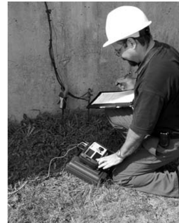
Using ART method with Megger DET3TC to test commercial ground without disconnecting the system
