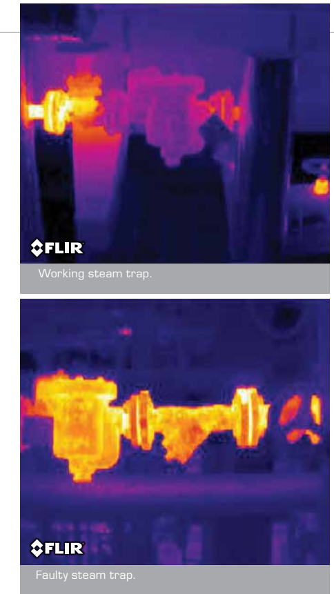
Energy Loss Discover missing insulation, faulty HVAC systems, and other issues that waste energy and lots of money.
