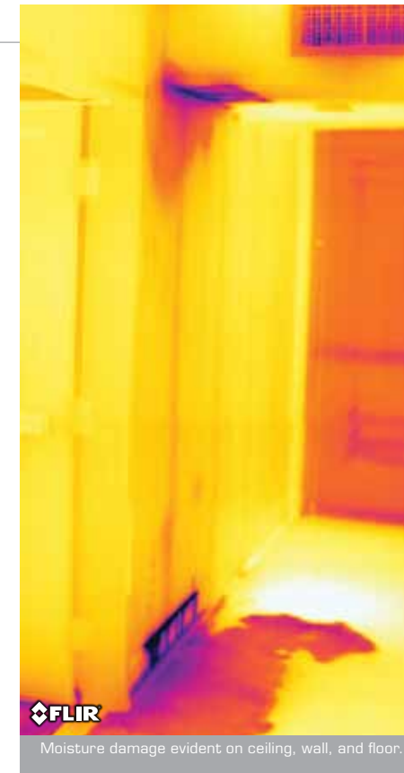
Building Diagnostics Even small areas of moisture intrusion can be easy to spot with an infrared camera. Locate and repair hidden water damage before a trickle turns into a flood.
