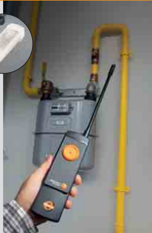
Checks for leaks in domestic gas pipes
