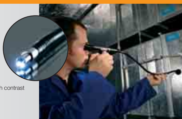
Inspects air duct, with gooseneck casing, middle flexibility
