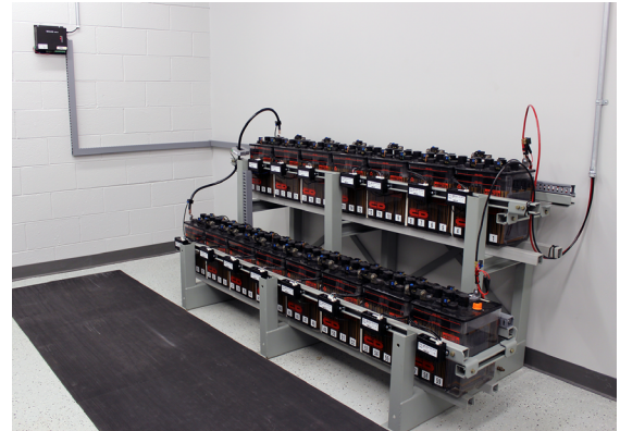
BQMS Installation on 125VDC Utility Battery System
