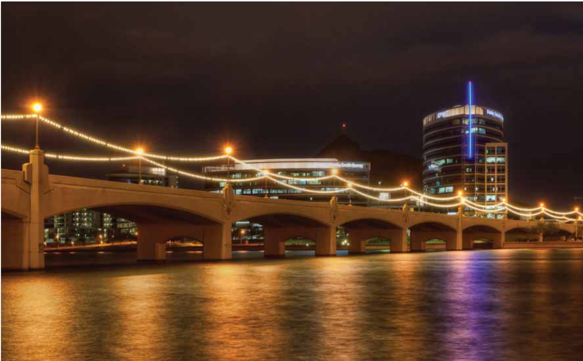
Application: Ericson stringlights (custom 12/3 black Navy Drop) light up bridge in Tempe, Arizona.
