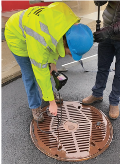
Figure 8.1 Inserting the probe into the test area.
