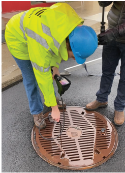
Figure 8.1 Inserting the probe into the test area.
