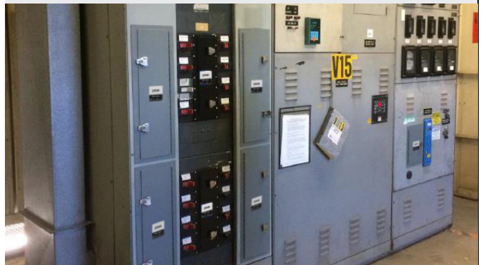
Final installation of the IR windows
