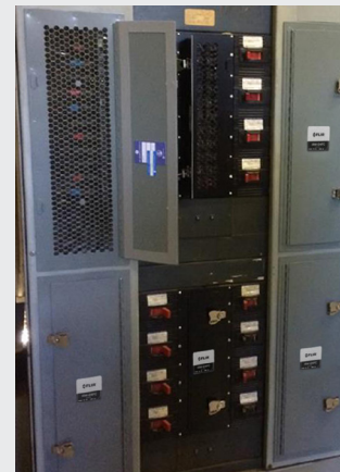
24-inch IR window installed at SLAC
