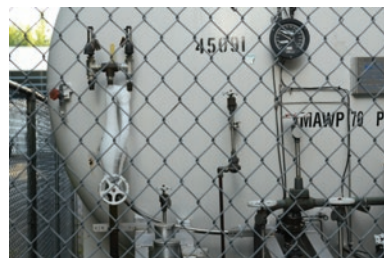
Difficult inspection sites
