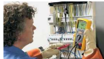
Insulation test at a distribution panel
