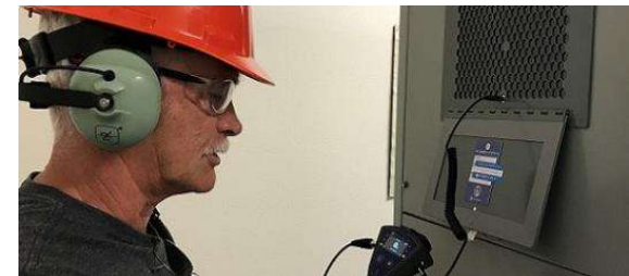
PD inspection through "ultrasonic window"
