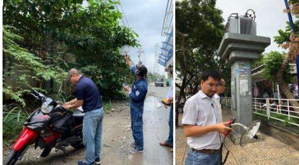
Routes across the city to inspect distribution lines, cabinets & transformers using ultrasound
