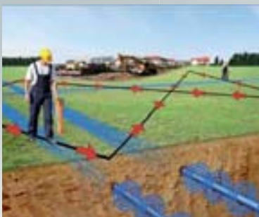
Use of meter for tracing of metallic conductors/pipes on a site planned for construction (e.g. excavation work)
