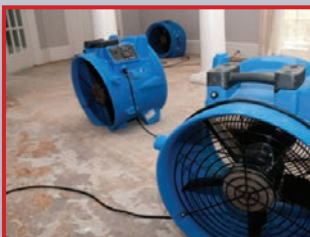
Monitor the drying part of water damage restoration
