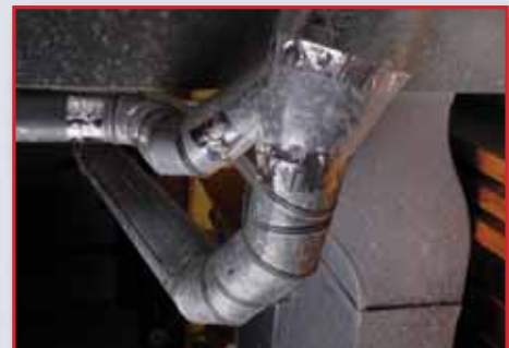
Minimally Invasive Duct Leak Testing
