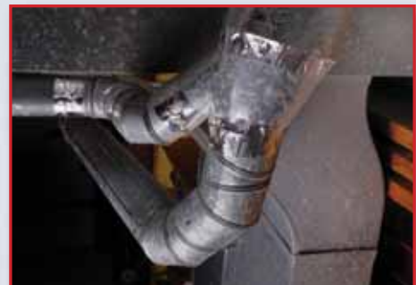
Minimally Invasive Duct Leak Testing
