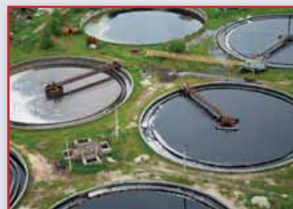
Water Pollution Control
