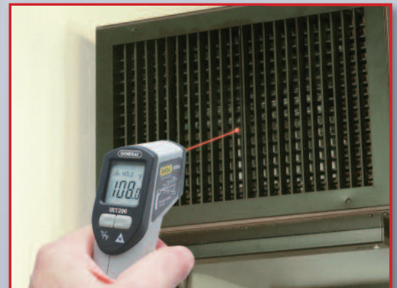
Performance-testing a new A/C system
