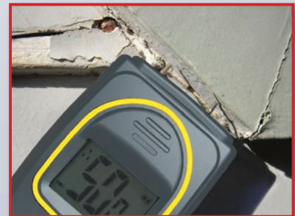
Check drywall for moisture
