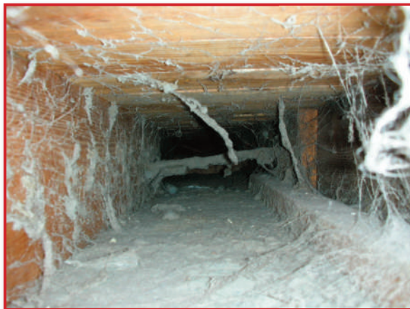
The VGA probes' four forward-facing LEDs and two rear-facing LEDs make the darkest crawl space as bright as day
