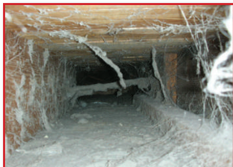
Inspection of hard-to-reach and hard-to-see areas
