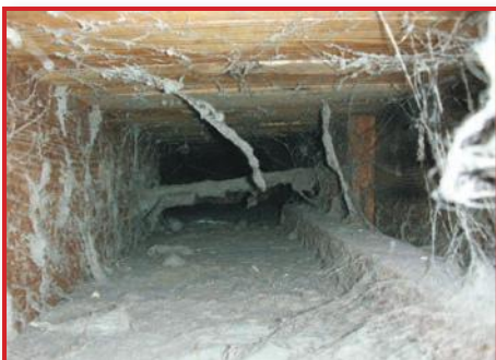
Inspection of hard-to-reach and hard-to-see areas
