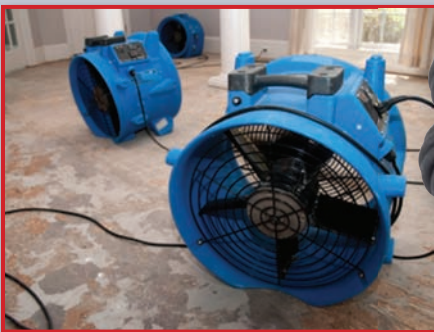
Check ambient temperature and humidity during restoration drying
