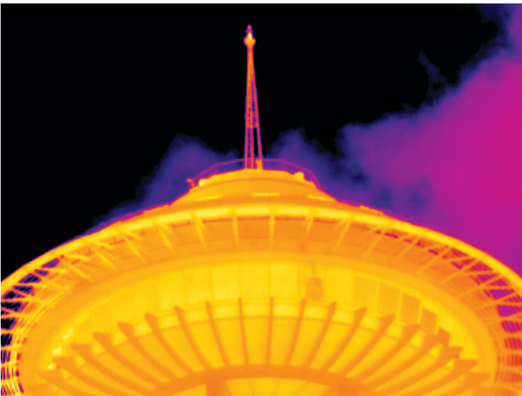
Figure 3: This third image was captured with a TiX560 infrared camera from the same location, with a Fluke 4x telephoto infrared lens.
