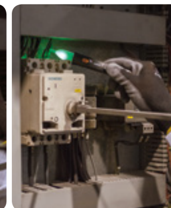
Step3 - If the green LED turns on with steady light, phase sequence is correct . If, however, the red LED flashes, phase sequence is incorrect .
