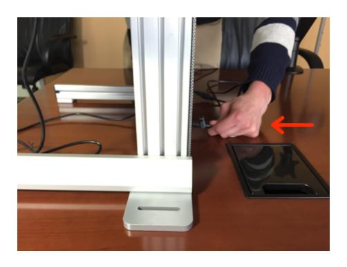
**Step 12** With the unit placed securely on the desk, lower work surface (G) over brackets.
