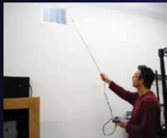
HVAC testing and balancing
