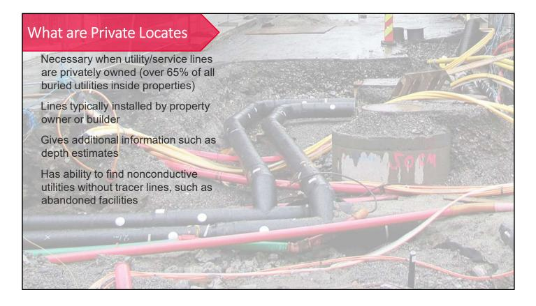
Private locates cover all utilities which need to be located. This work typically utilizes EML and also GPR. They will do all they can to locate the utilities within the excavation area. They will supply depth measurements where possible and also have the ability to documents. The technology we have in Leica allows the contract to perform these tasks himself, quickly and simply.
