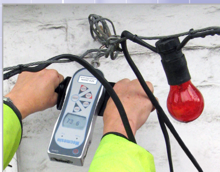
Pull test on anchorage points
