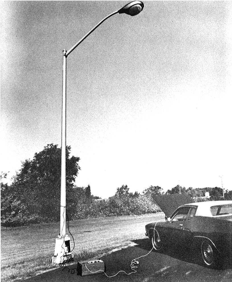
Figure 8: Testing Parking Lot Lighting; the Test Set Shown is Operating from an Inverter
