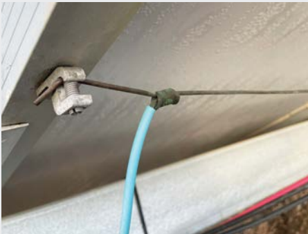
Figures 6-2 and 6-3: Left—Dubious bonding. Right—A lay-in lug bonds listed PV racking to the equipment grounding conductor.
