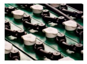
This creates a problem when testing batteries. In order to perform proper measurements of battery cell impedance, inter-cell connection resistance (straps) and terminal resistance, the measurement needs to be made on the post of the battery.
