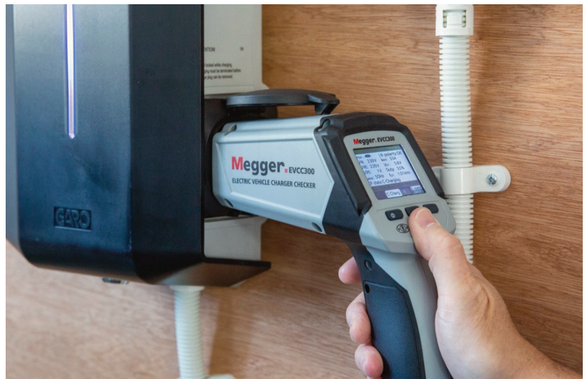
Periodic Testing of an Installed Charge Point
