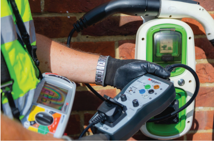
Testing a New Charge Point Installation
