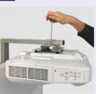
Attach the projector to the arm and tighten the screws.
