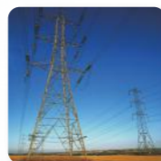
Electric Power Engineering
