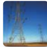
Electric Power Engineering
