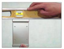
2. Use a level to determine the proper level of the CRS201.
