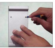
3. Mark the four screw holes on the bracket with a pencil.
